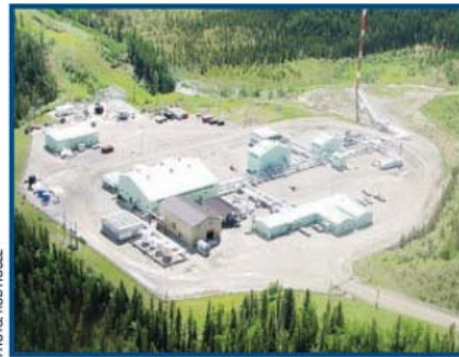
FireSmart Industrial Zone 1: 0-10 metres from structure(s) on the disposition. (Priority One - personnel and structures are at risk from radiant heat and ember transport associated with a wildfire.)
